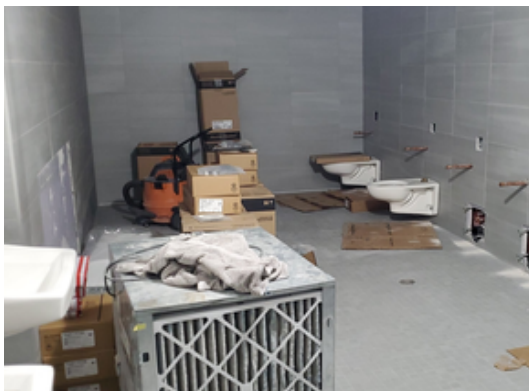
Middle School – Third Level Restroom Tile and Plumbing Fixtures Installation
