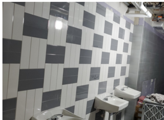
Middle School – Third Level Restroom Tile and Plumbing Fixtures Installation
